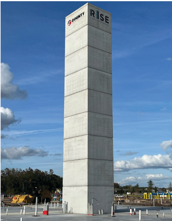
Elevator Shaft
