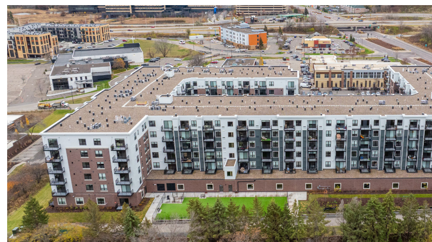
A completed podium construction project showcases how a precast concrete podium supports upper-level residential floors, delivering durability, fire resistance, and efficient use of space in mid-rise multifamily developments.
