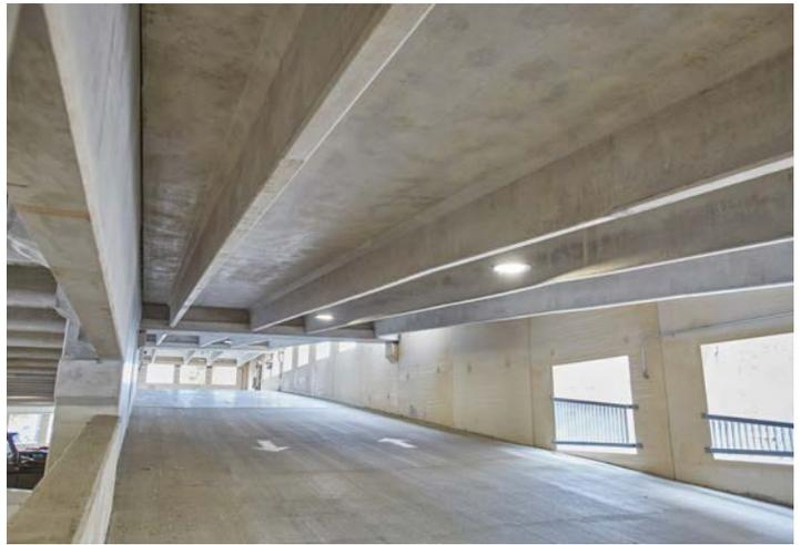
To seamlessly integrate the parking structure into its historic downtown surroundings, County Prestress manufactured beige spandrels, wall panels, and exterior columns and concrete brick infills. These components protect and visually enhance the structure.
