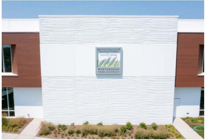
Architectural panels were produced with form liners that enhanced the aesthetic appeal of the activity center's façade. From reproducing textures found in nature, like wood grains and stacked rocks, to custom artistic patterns, form liners demonstrate the design flexibility of precast concrete.
